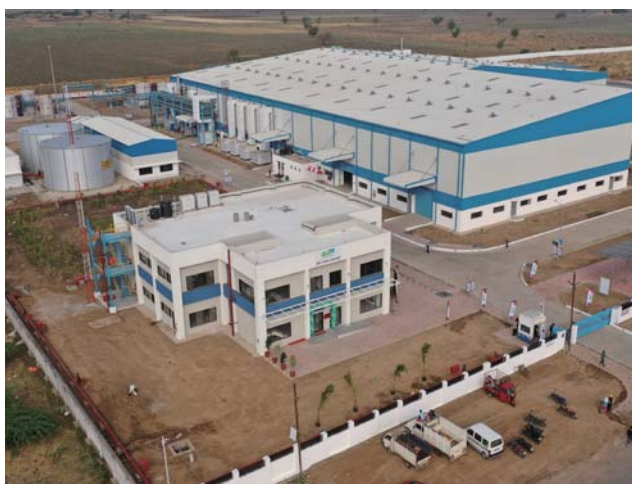
Printing inks production facility (India)
