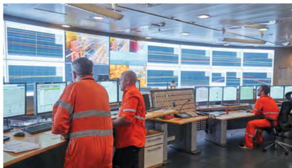
Control center inside the CPF
