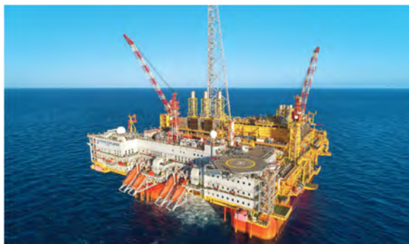
Offshore production and central processing facility (CPF)
