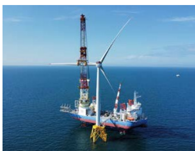
Ishikari Bay New Port Offshore Windfarm (SEP vessel)
